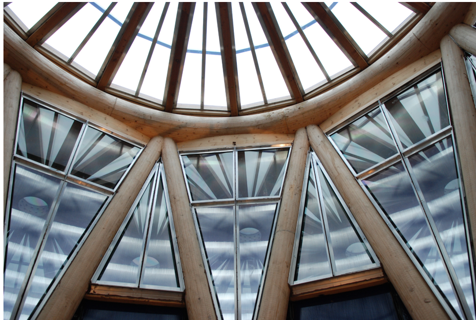
Figure 7: The SPD Smart Glass skylight inside the Globe of Science and Innovation
